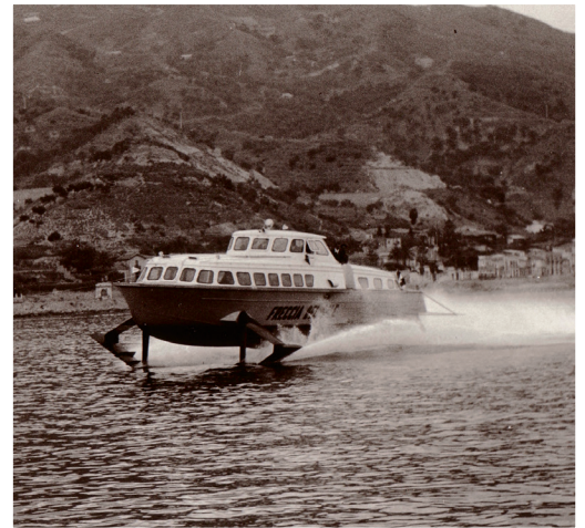
Above, the first commercial Hydrofoil "Freccia del Sole"
